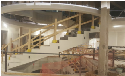
Site ready for scan
